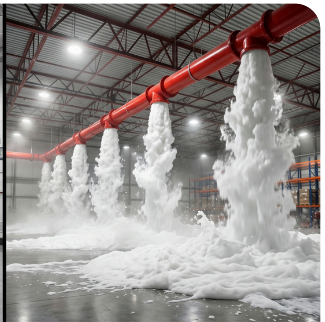
FOAM FLOODING SYSTEM
