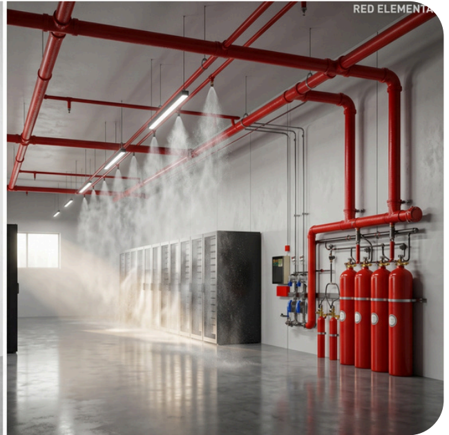
TOTAL FLOODING SYSTEM
