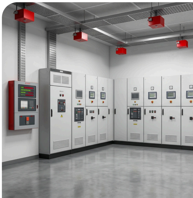
AEROSOL SUPPRESSION SYSTEM
